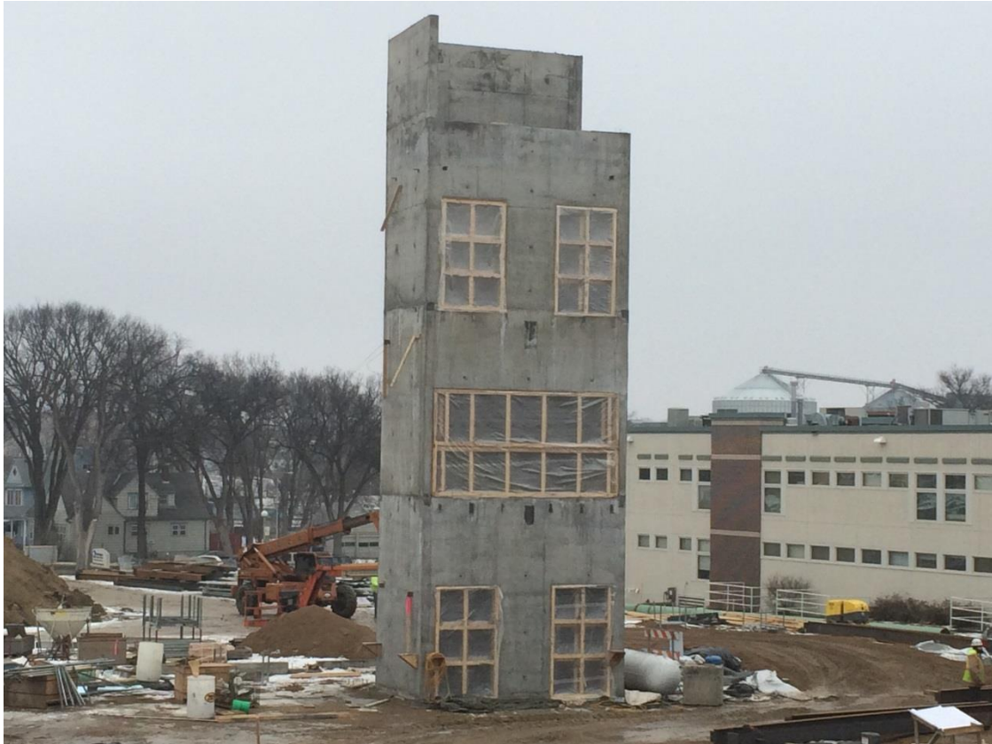
Elevator core walls complete.
