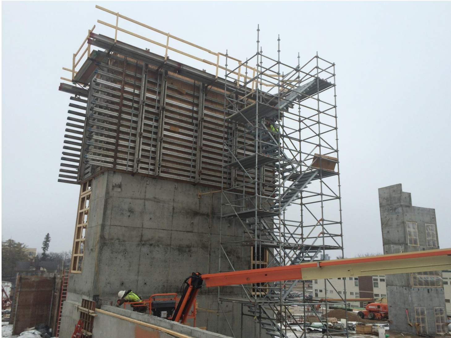
Third and final level of Stair A being formed.
