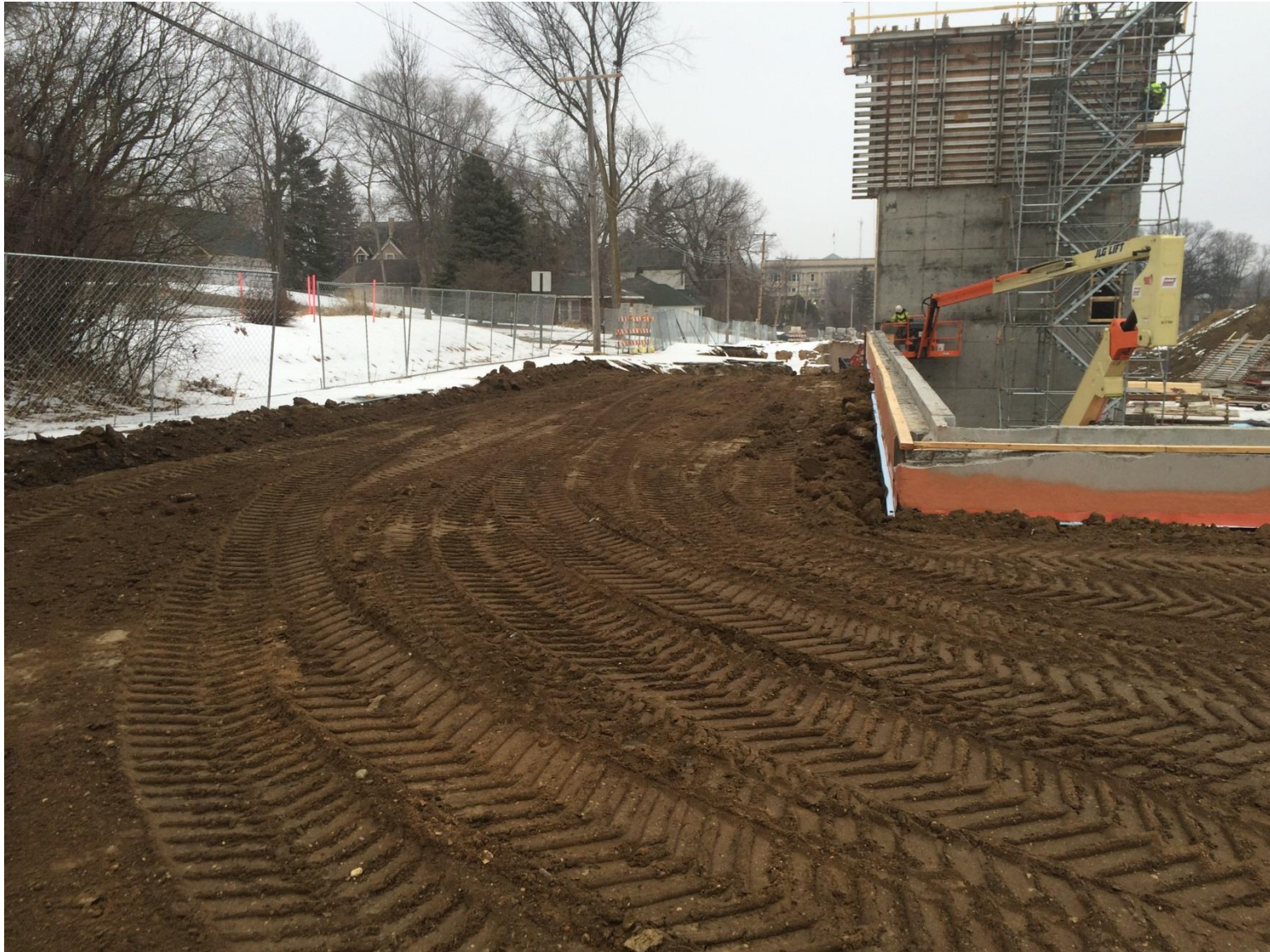
West wall water proofed and backfilled.
